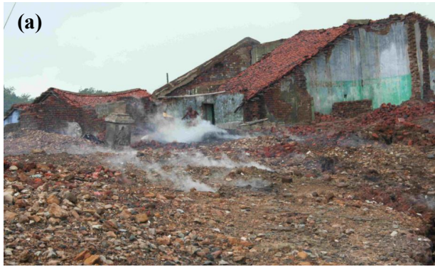
Fig.2.7.4. a,b: Huts damaged due to subsidence related to coal fire in Kendwadiah village
