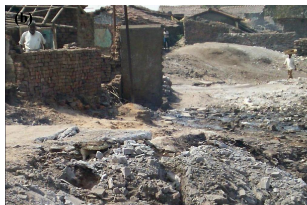
Fig.2.7.6. a: Hutments damaged (demolished) in Kusunda area due to subsidence b: Land subsidence in Bokapahari due to advancing fire
