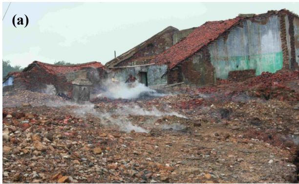
Fig. 2.7.7(a),(b): Huts damaged due to subsidence related to fire in Kendwadih village
