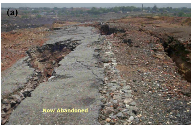
Fig. 2.7.9 (a): Cracks/fissure development in the main road in East Katras due to fire (now abandoned) (b): fissure development in Gwala basti (E.ast Bassuriya)
