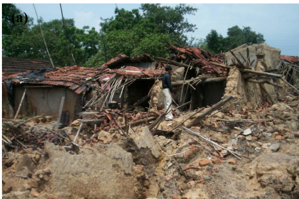
Fig.2.7.6. a: Hutments damaged (demolished) in Kusunda area due to subsidence b: Land subsidence in Bokapahari due to advancing fire
