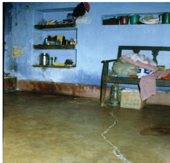
Fig.2.7.5.: Cracks developed in the floor of a house in Ena-Islampur due to coal fire
