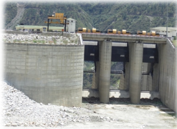
Slide gates of main dam structure
