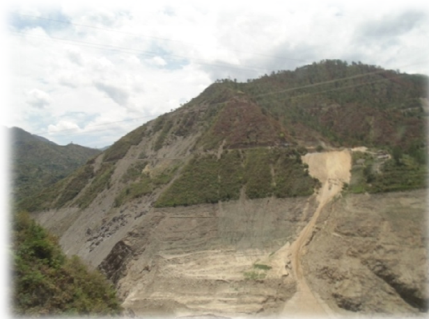
Toe erosion and Landslide along the vicinity of the dam
