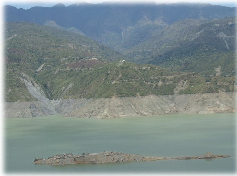
Submerged Tehri town and toe erosion along the reservoir
