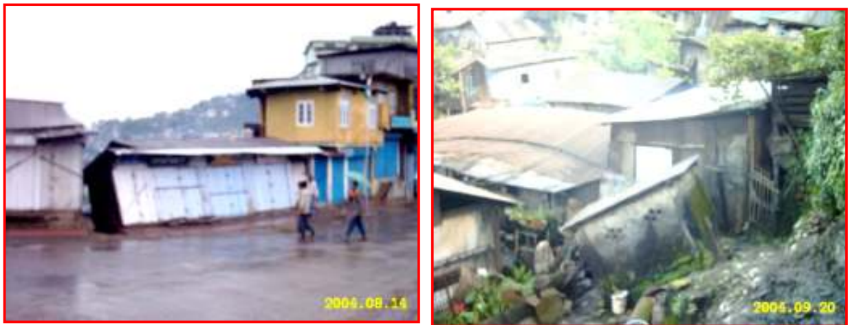
Figure 3.3.3: Photographs showing Buildings affected by Creeping Slides
