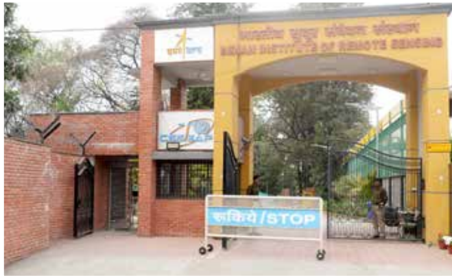
Main Gate (Outside View)
