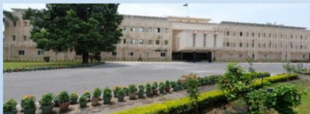
IIRS Main Building
