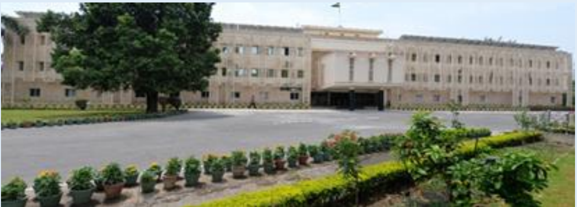
Fig. 1. IIRS Main Building
