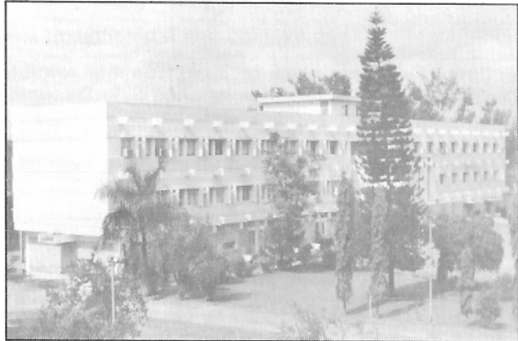
IIRS Main Building
