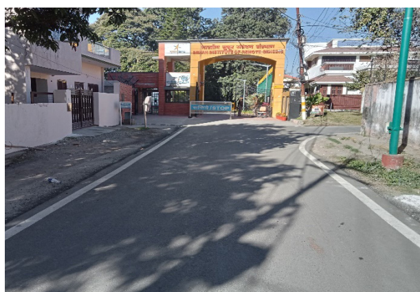
New bituminous surface repair of approach road
