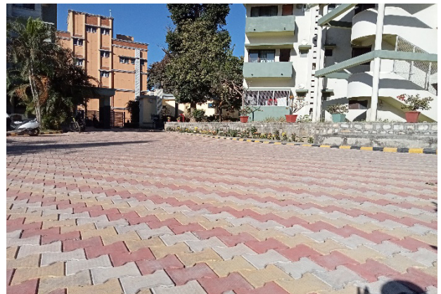
New paver block road in front of International Hostel
